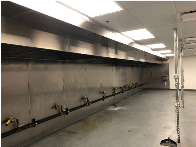
Exhaust Hood with Fire Protection
