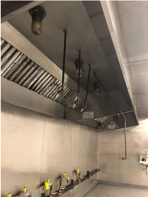
Exhaust Hood with Fire Protection
