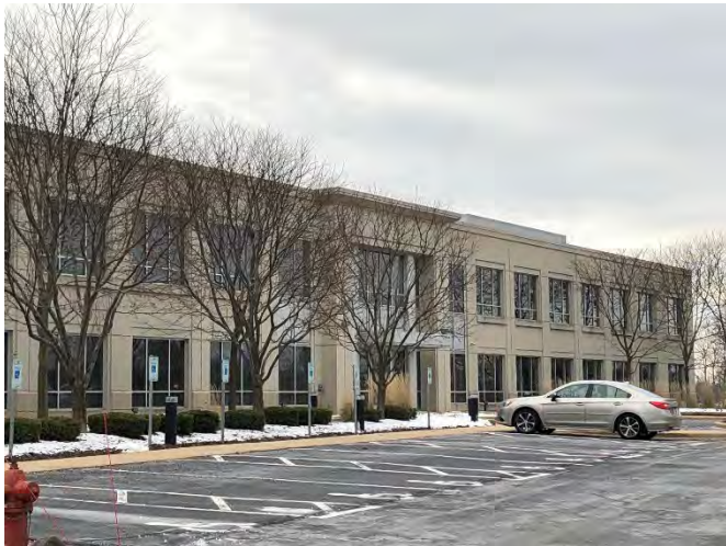
8 Handicap Stalls at Main Entry
