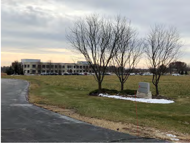
North Service Drive Entrance
