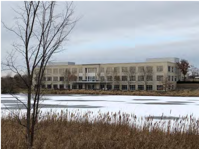
View from Hwy 36
