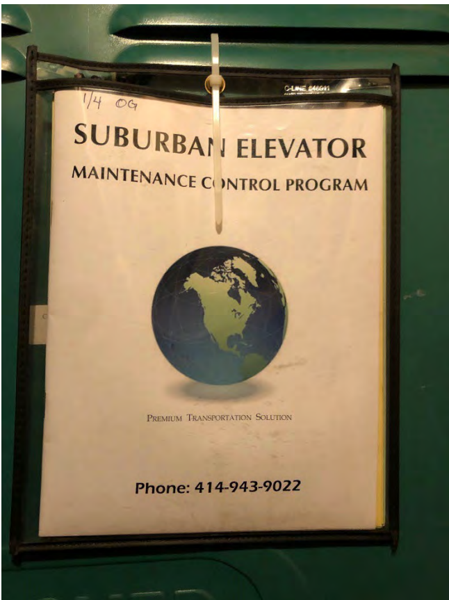
Properly maintained hydraulic elevator
