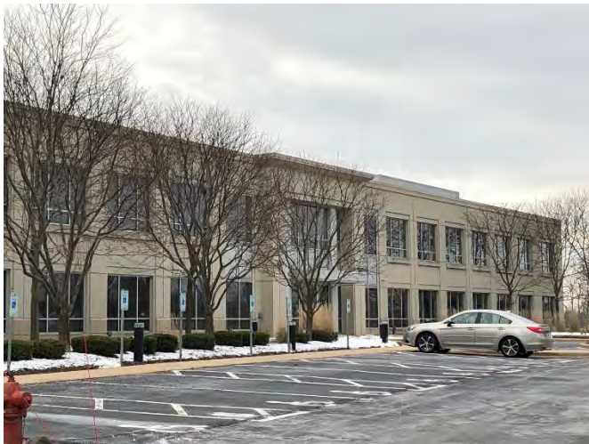
8 Handicap Stalls at Main Entry
