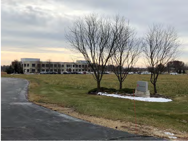
North Service Drive Entrance
